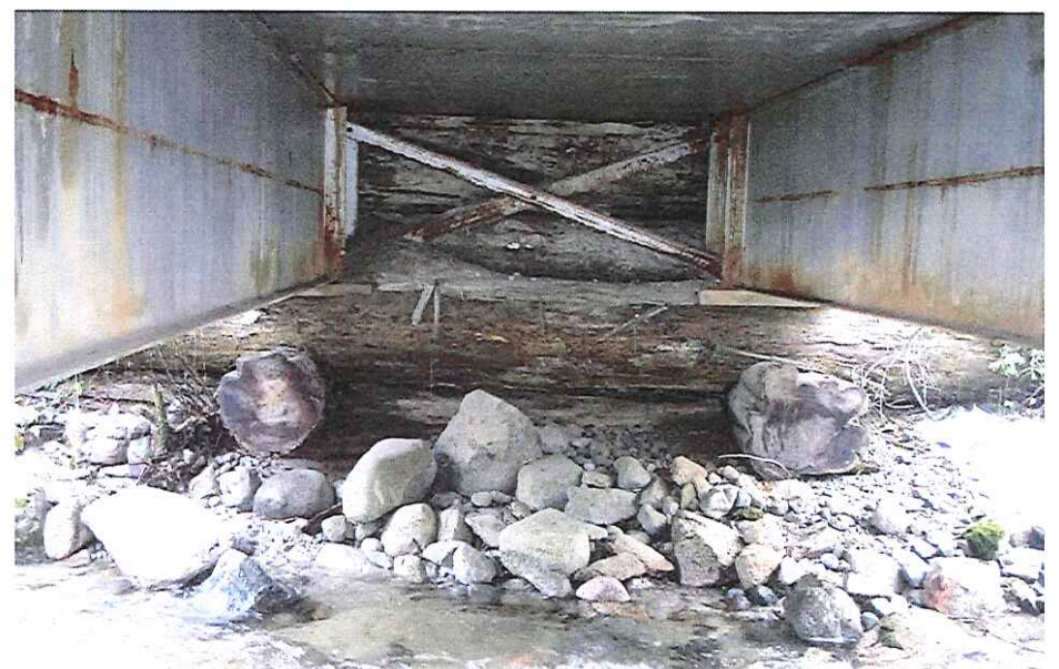
CK-2020Abutment Right Bank
