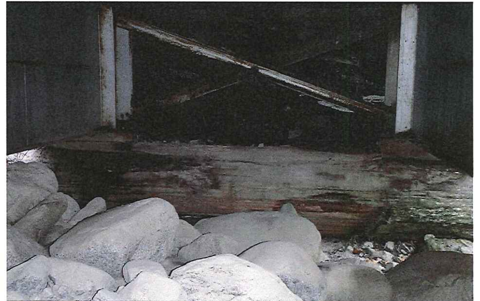
CK-2020Abutment Left Bank
