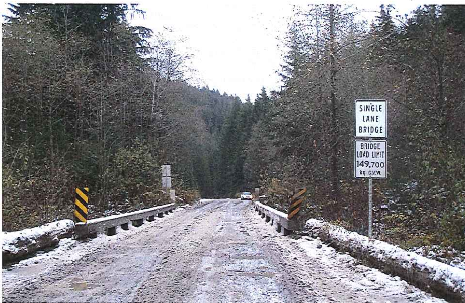
CK-2020Approach Right Bank
